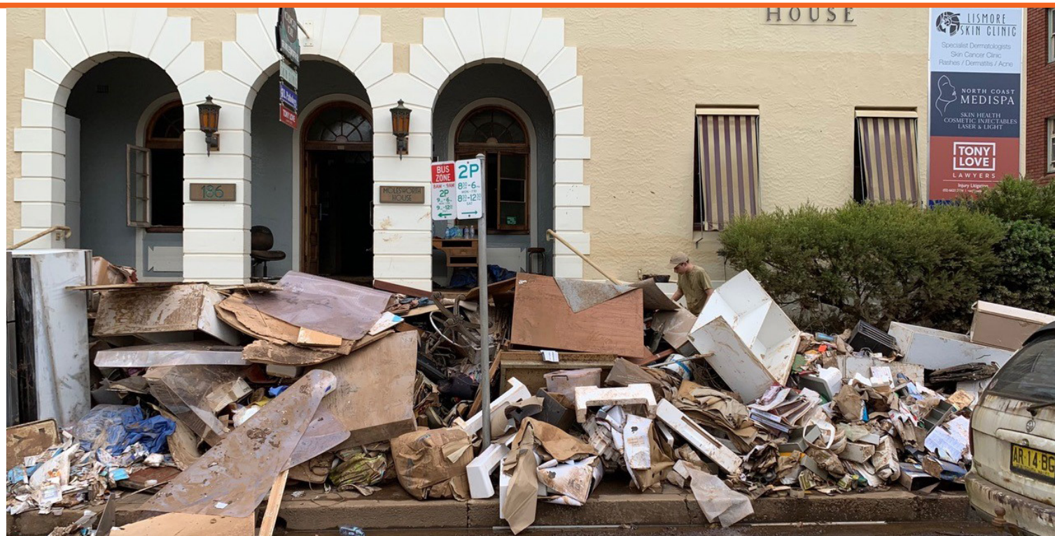
Floodwaters damaged the Lismore Skin Clinic.
